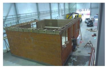
Fig.6 – Erection of the VUKONZE Climate chamber envelope.
