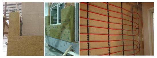
Fig.8 – Details of the VUKONZE Climate chamber additional insulation and wall heating system.
